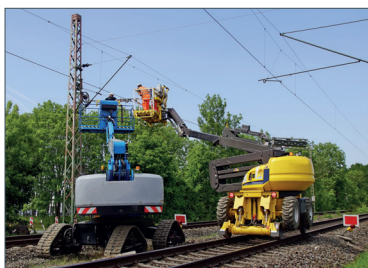
Construction of contact lines
