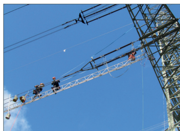
Overhead line construction
