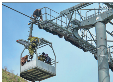
Cable car construction
